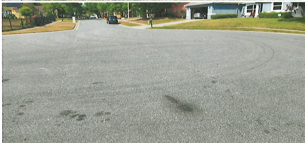
Pictures 1-5: Dock, Sidewalks, and Curbing around Cul-de-Sac. Lake near Johio Shores/New Victor Road entrance to Waterside subdivision.
