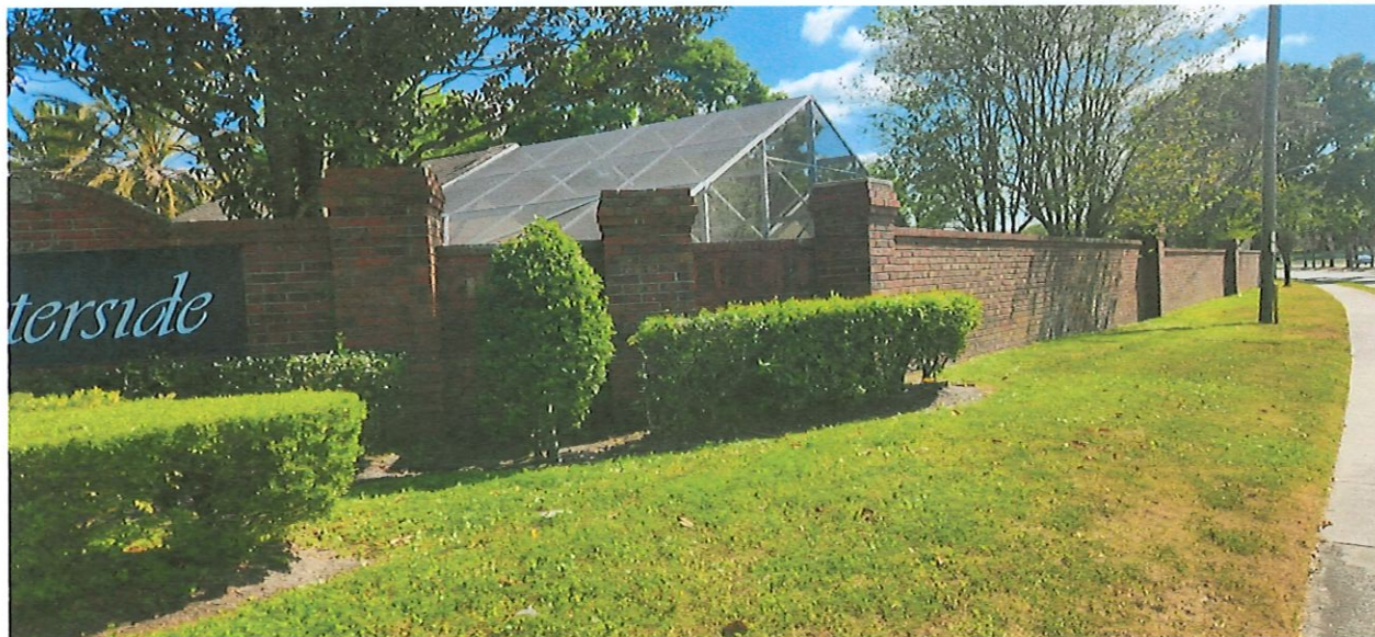
Picture 7 Above: Monument Sign on Clarke Rd and New Victor (south) and Brick Wall
