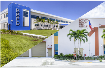
City of Boynton Beach Police Dept. HQ & Fire Station 1
