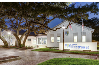
Town of Windermere Police Department & Town Facilities
