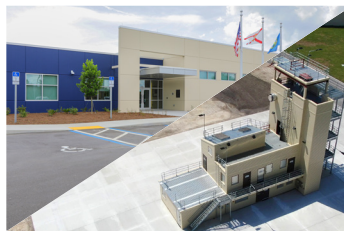
City of Kissimmee Public Safety Training Facility & Fire Tower
