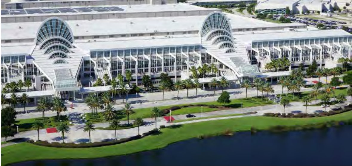
FIGURE 1: A REPRESENTATIVE PROJECT, ORANGE COUNTY CONVENTION CENTER
