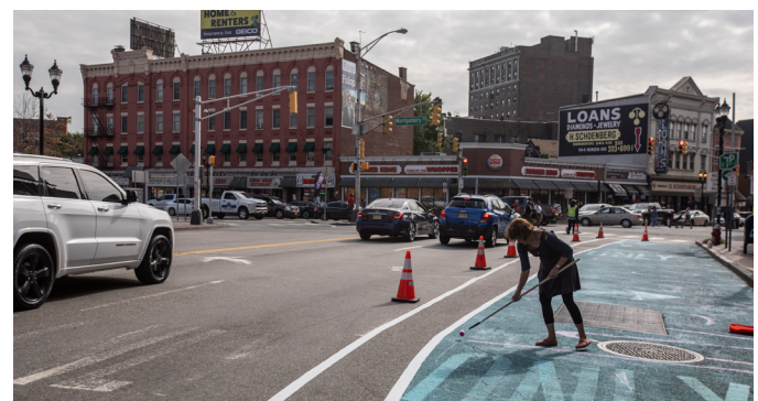
Figure 15. Volunteers helped paint over an exclusive right turn lane as part of a demonstration project to improve the safety of the corridor for bicyclists and pedestrians (above); inexpensive but more permanent treatments were installed as a result of the demonstration project’s success (left) (City of Jersey City)
