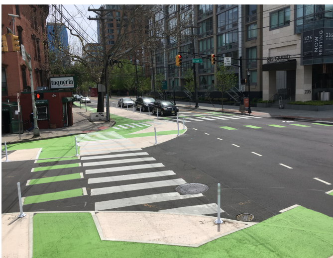
Figure 16. Paint and flexible delineators were used to quickly create Jersey City’s first protected intersection connecting two protected bike lane paths (City of Jersey City)
