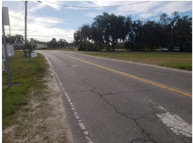
Looking south along Taylor Street from near the northwest corner of the site (subject on left)
