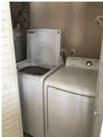
Utility Closet in Kitchen
